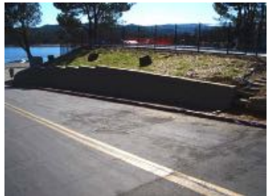
New Retaining Wall below Pool Built by Volunteers
