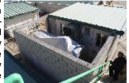
New Back-up Generator Under Construction
